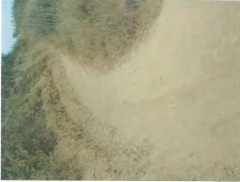
The above photo demonstrates the trenching that can occur when a trail characterized by dry, powdery soil sees considerable use by mountain bikers. July 2009
